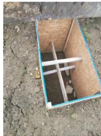
The hole for the foundation is dug and the form is in.
